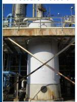
5004 15,700 Gallon vertical 304L-SS Tank. Internal Rated 50 PSI @ 225 deg F. Dished heads. 11' dia x 20' T/T (OAL - 27'). Shell thickness: 0.25", Head thickness: 0.375". Skirt mounted. Built by James Machine Works, 1996, S/N: 6673, NB# 2317. Approx Wt: 20,000 lbs. Previous use: Ketazine Col. Feed Tank.
